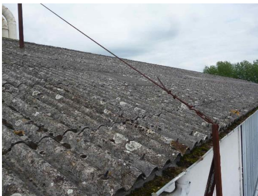
P32 – Chaufferie, hangar 2-3-4
